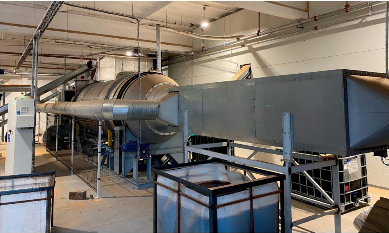
/ 2. Recuperator that recovers 200 kW of heat at a temperature of 170°C
